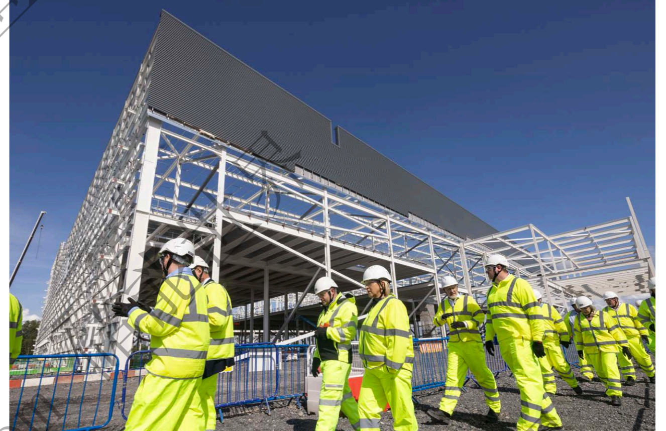
Agratas gigafactory, Bridgwater, Somerset, October 2025
