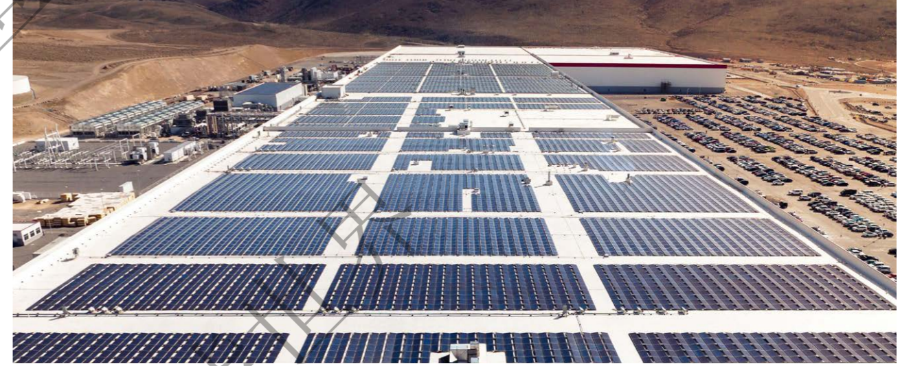
Solar panels on the roof of a gigafactory
