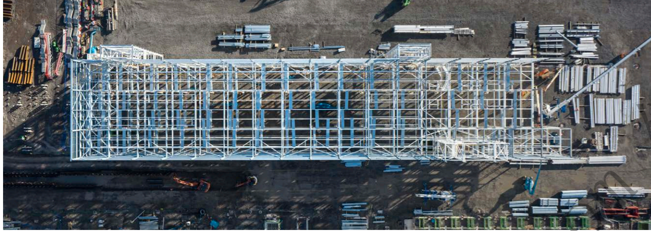
Agratas site, Bridgwater, Somerset, November 2025
